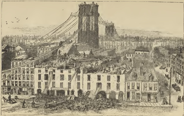
TEARING DOWN BUILDINGS FOR APPROACHES TO BROOKLYN BRIDGE.
